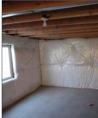
Fiberglass batt w/ vinyl backing
